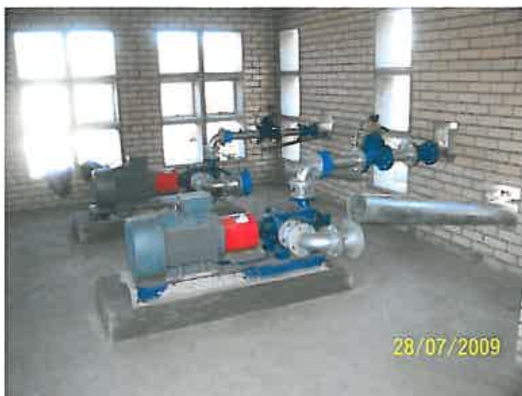
Coronation/Enyathi – Water treatment works: Filter pumps
