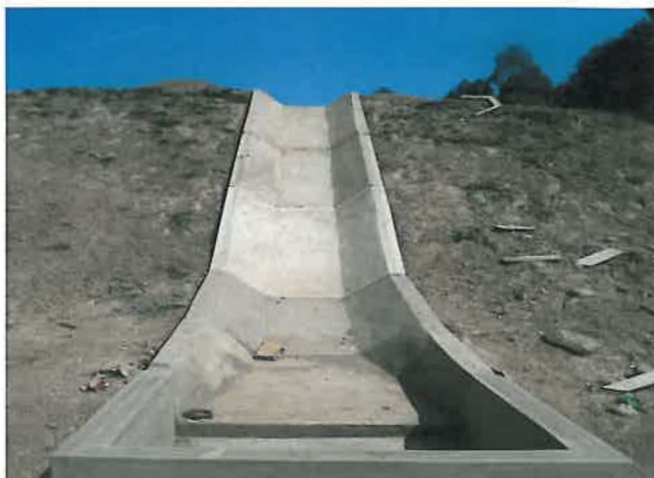
Coronation/Enyathi – Waste Water treatment works : Sewer pond emergency overflow
