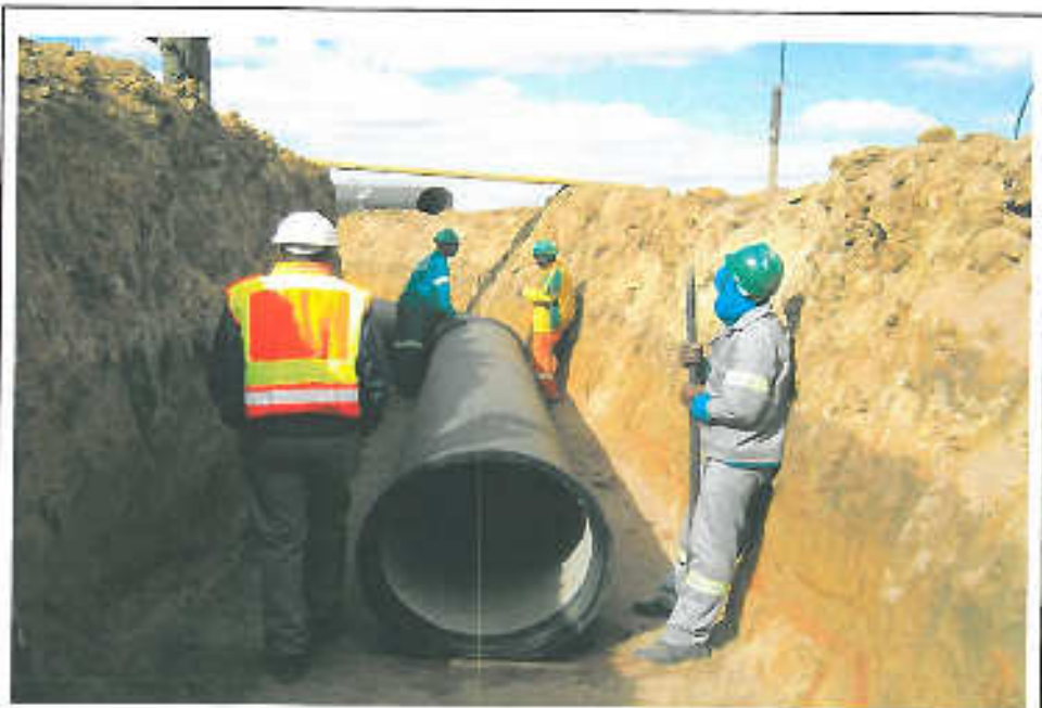
A R20M KLIPFONTEIN RISING MAIN PROJECT
